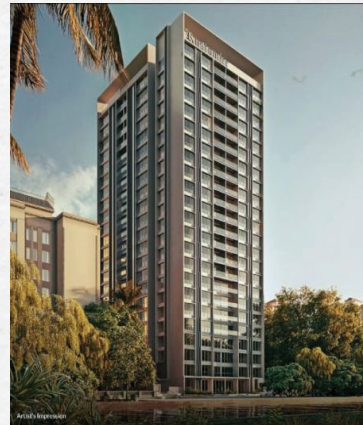
Rustomjee Reserve Mumbai 22 Storey High Rise Tower
